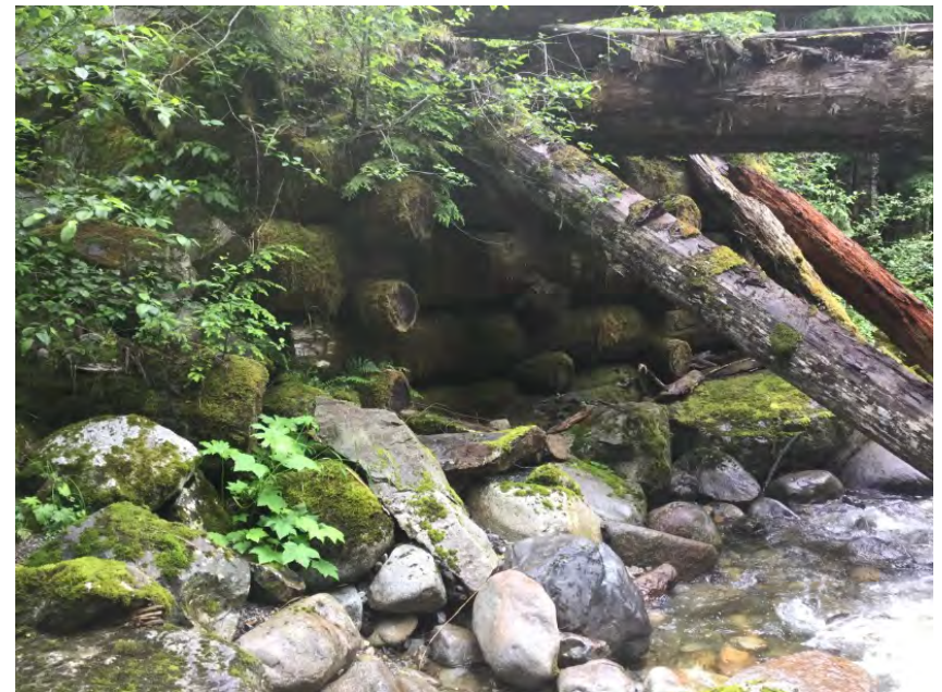
Left Bank Abutment when facing downstream
