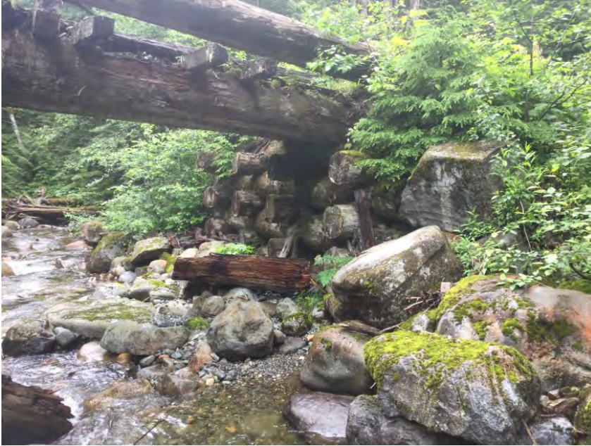
Right Bank Abutment when facing downstream
